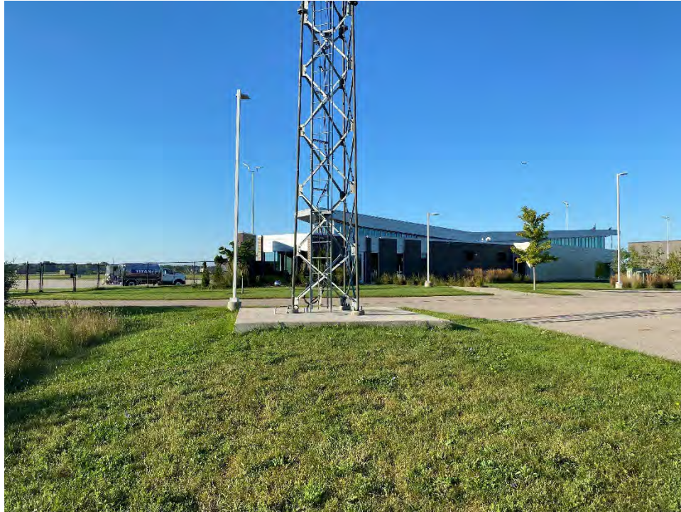
Photo 9. Recently constructed airport facility, facing southwest
