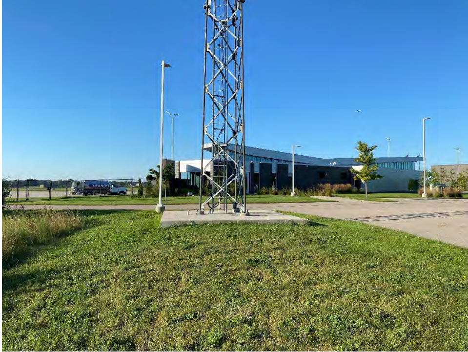
Photo 9. Recently constructed airport facility, facing southwest
