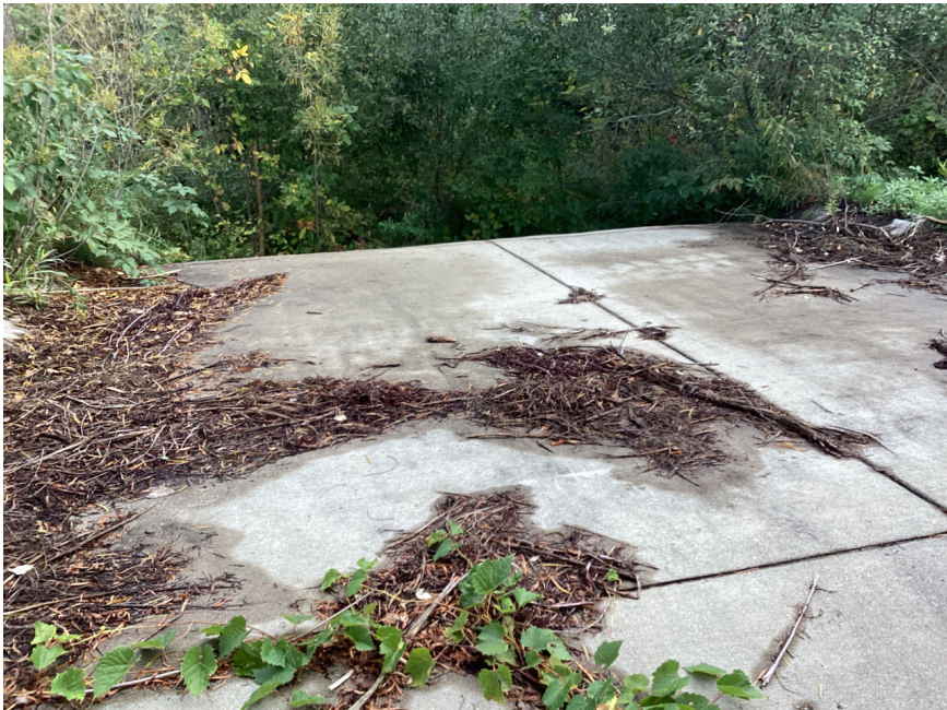
Photo 18. Weir at Wetland 3. View to the northeast.
