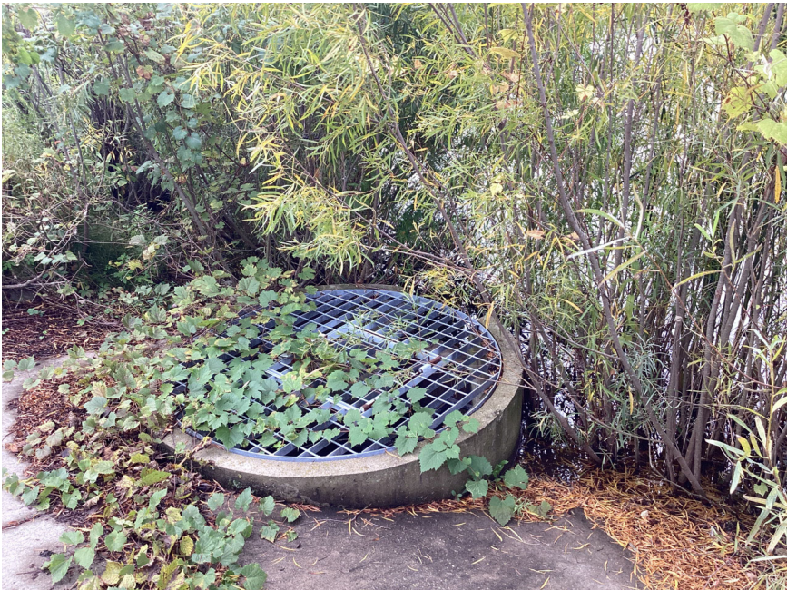
Photo 17. Overflow structure at Wetland 3. View to the south.
