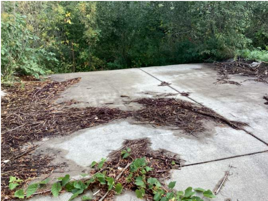
Photo 18. Weir at Wetland 3. View to the northeast.
